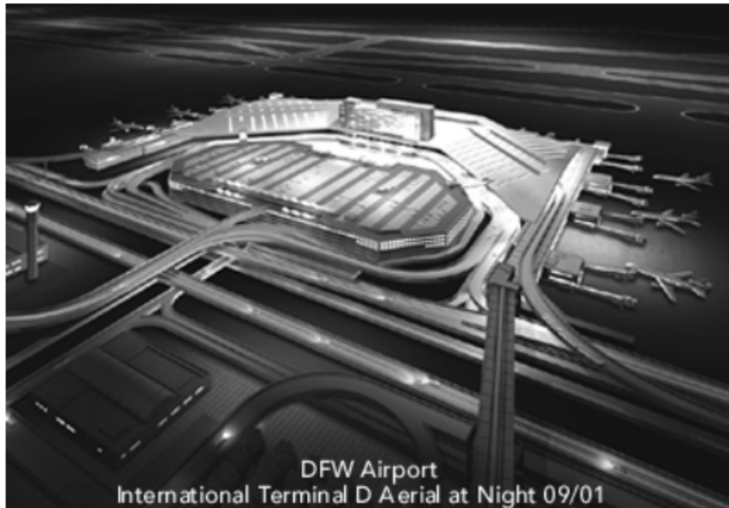
Figure 5.24: Dallas Fort worth International Airport – Terminal D Design Source : Dallas Fort worth International Airport, retrieved August 18 2002 from http://www.dfwairport.com/cdp/terminal_d.htm
